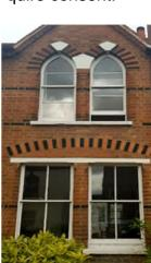
Fig.72 19 Mill Lane, Victorian sash windows, with larger panes
