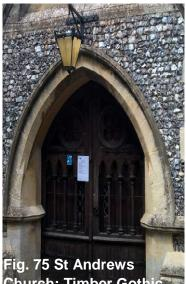
Fig. 75 St Andrews Church: Timber Gothic stye door with tracery detailing
