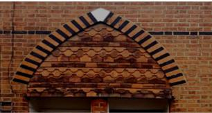
Fig. 59 bull nose and fishtail pattern tile hanging, and decorative brick and stonework detailing on one of the Victorian terraces
