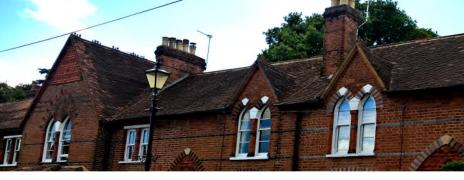
Fig .68 15-35 Mill Lane, gables and chimneys with terracotta chimney pots
